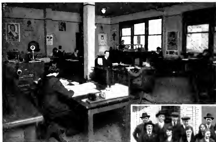
Main Office Des Moines Exchange
